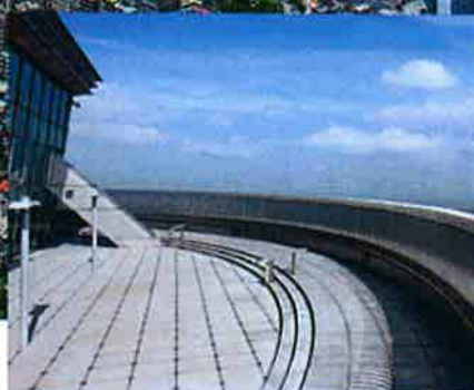
91樓戶外觀景觀 91F Outdoor Observatory
